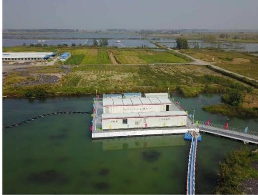
**Figure 3.** Completed Floating Switch Station on Water
